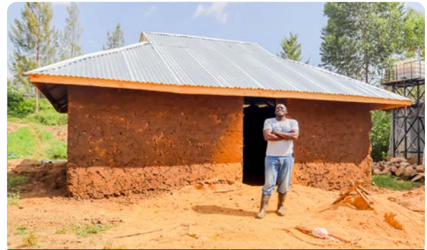
A proud Christopher poses in front of his ongoing house construction project Photo: Hydro Victoria/ Anne Nasumba.
