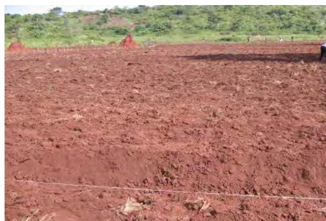
Field marking using strings
