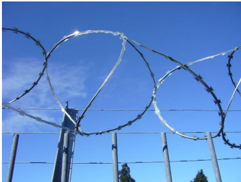
Razor wire reinforcement on top of poles.
